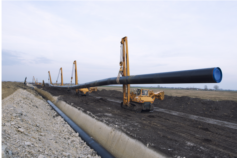
Figure 1.1: Placement of circular pipes for gas transportation.
