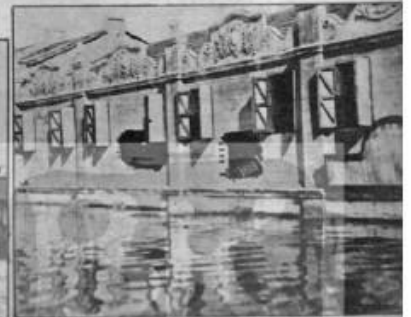
(攝英黃) 出逃壁穿民居樓上淹水 Holes made in walls for escape when water is rising up to the upper story
