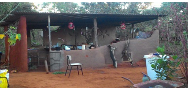
Figures 130 and 131: Kitchen built of clay and reused woods and Chaya to replace cabbage. Source: Acácio Machado.
