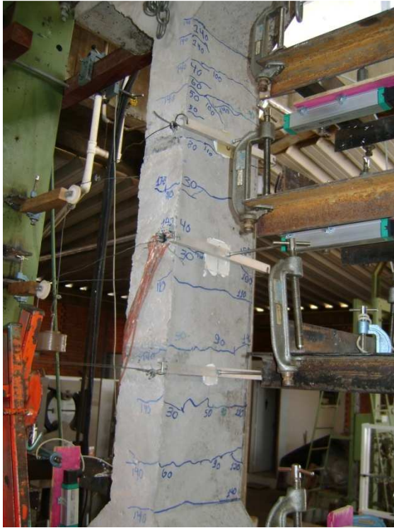
Figura 4.12-Fissuras no Pilar PFN 50 - 2,0
