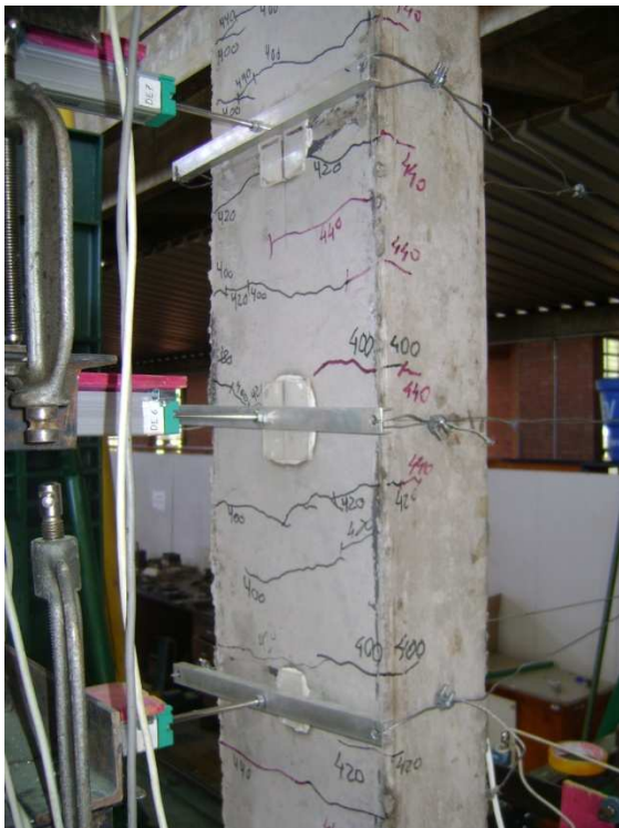
Figura 4.6 - Fissuras no Pilar PFN 24 - 2,0
