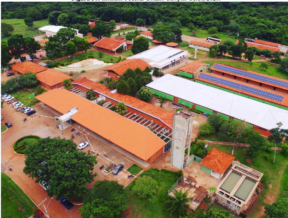
Figura 36: Instituto Federal Goiano Campus Ceres , 2020.
